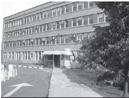
Community Services is located in the Jeffery Hale Pavilion
